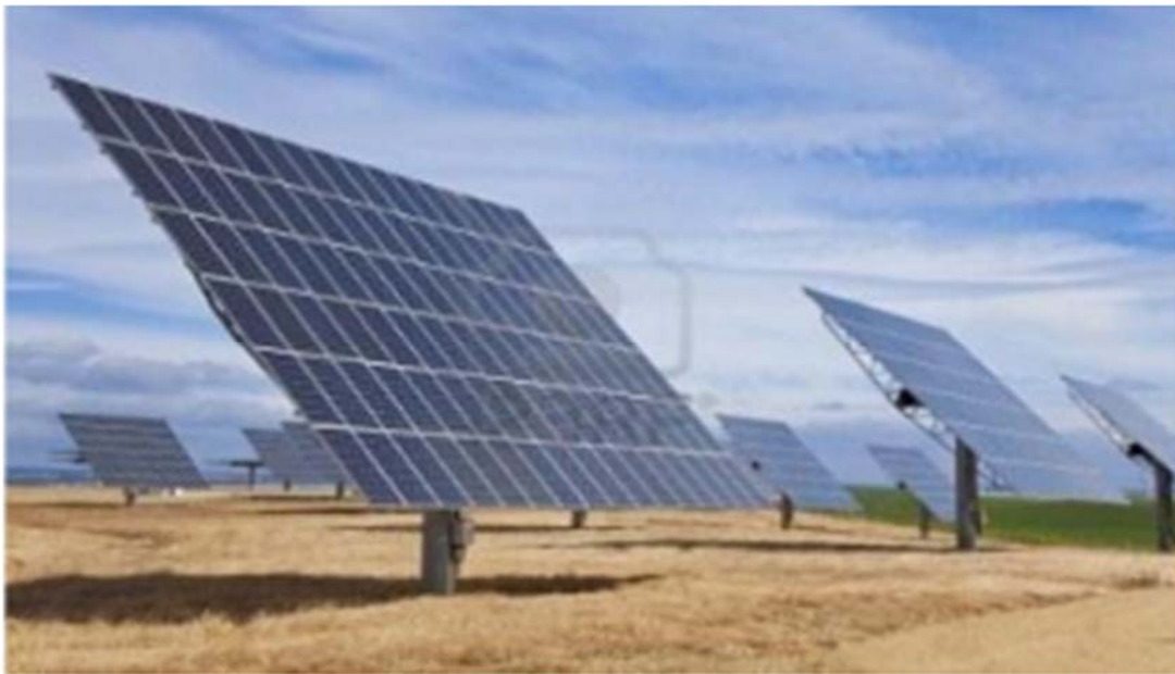
Figure 1: Represented the A square solar panel with two degrees of freedom is set up.
